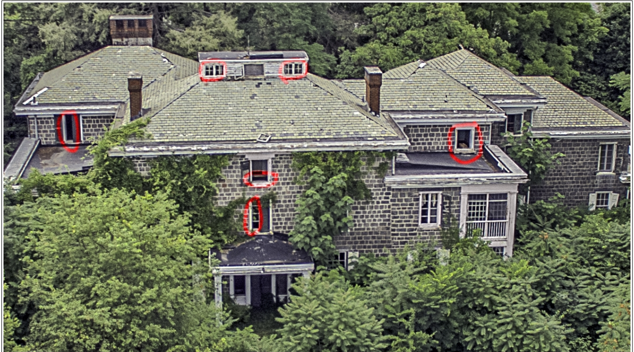
2016 07 03 Open windows, missing window panes. Missing roof tiles.
