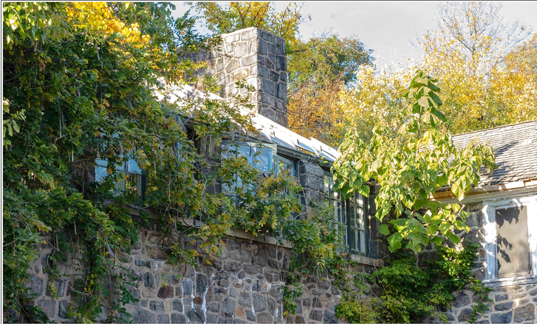
Gibraltar- Greenhouse Southern Facade #2 11 06 2021
